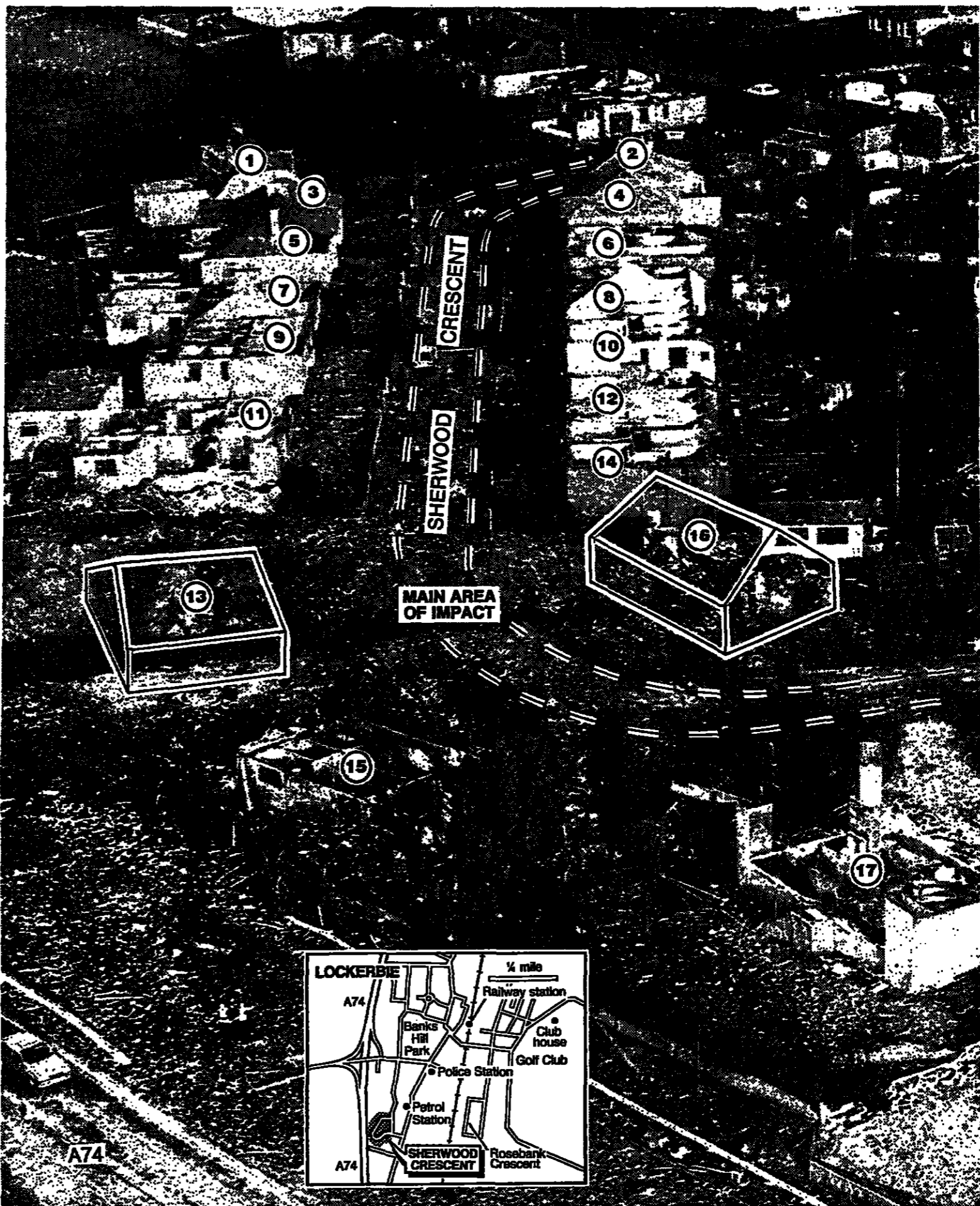
Sherwood Crescent: Some houses at the top end of the street appear relatively unscathed, but near the A74, little or nothing remains.
